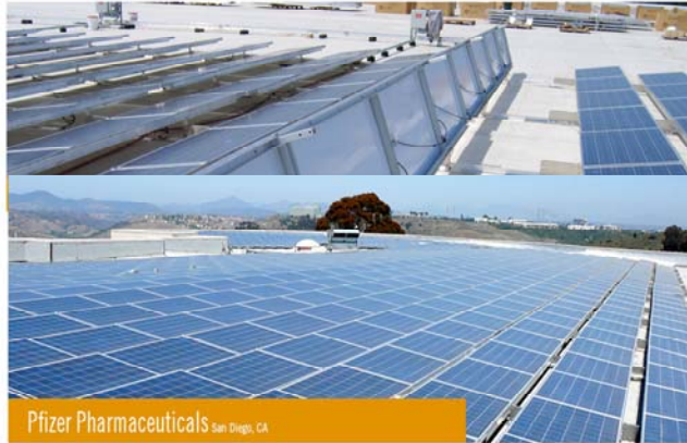
Pfizer = KW 337 Tilt Angle 5 deg. Number of Modules 1,372 Model Sharp
