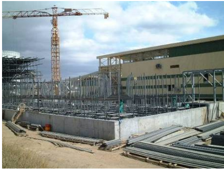
64 MW Olkaria II during construction – Kenya, 20904.
