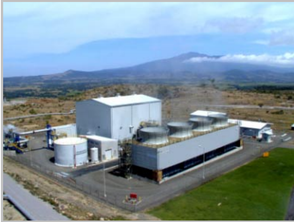
The Miravalles III Geothermal Project, Costa Rica
